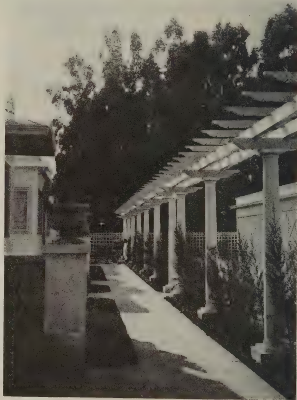
THE PERGOLA SEPARATING THE GARAGES FROM THE HOUSES.
